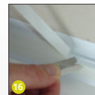
16 Apply masking tape to strip and trim off.
