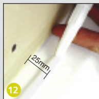
12 Lay silicone on ledge using finger as guide.
