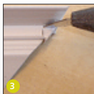
2 Notch mitred corners with sharp blade or snips as shown above.
