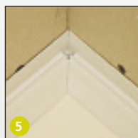
5 Dry fit to check corner joints meet.
