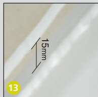
13 Lay silicone on wall approx 15mm above ledge.
