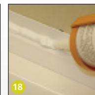
18 Lay Sealux-N on strip and install panel.
