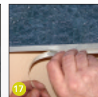
17 Apply masking tape to panel and trim off.
