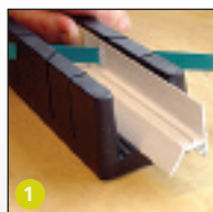
1 Measure & cut strip. Remove saw frays.
