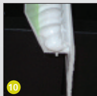
10 Lay silicone in strip in 400mm stages.
